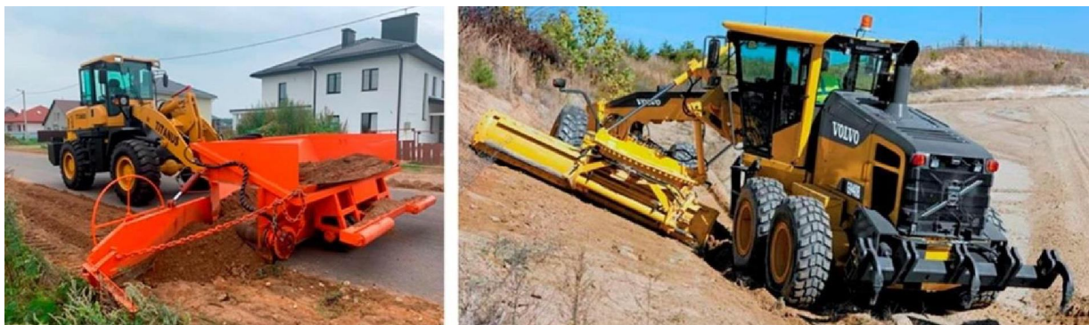
Figure 1 – Work during laying and widening of road shoulders
